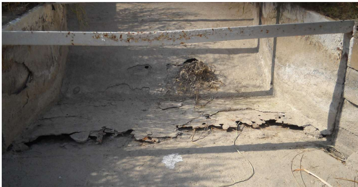
Figure 20. The Frontier Ditch flume, proposed to be replaced.
